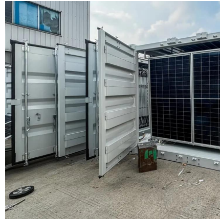
Containerized Battery Energy Storage System ...
