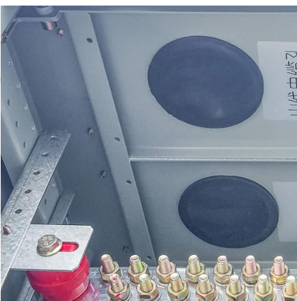
POWER PLANT PROFILE BRAZZAVILLE SOLAR PV PROJECT ...
