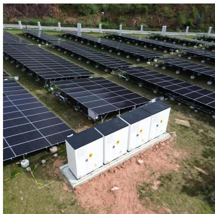
[5MWh Air-Cooled Container Energy Storage System](#)
