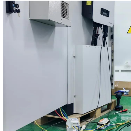
SmartGen HBMS100 Energy storage Battery cabinet
