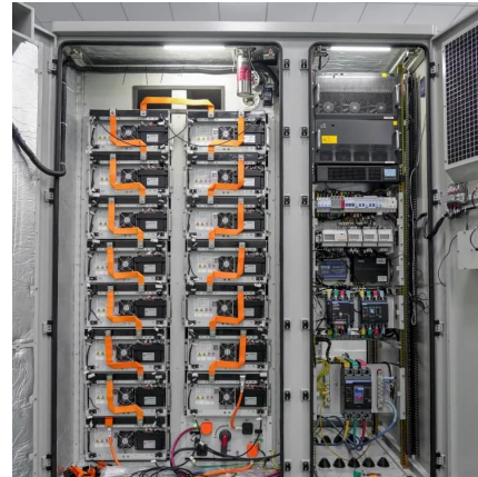
200kW Off Grid solar system (230.4kWh)
