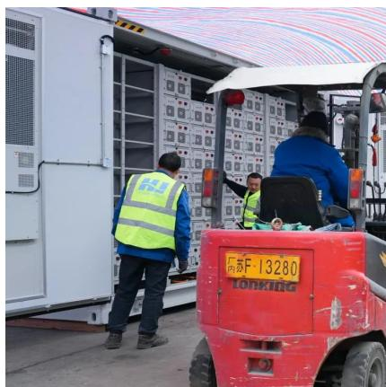
[Lithium iron phosphate battery energy storage container](#)
