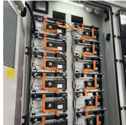
Solarcontainer: The mobile solar system
