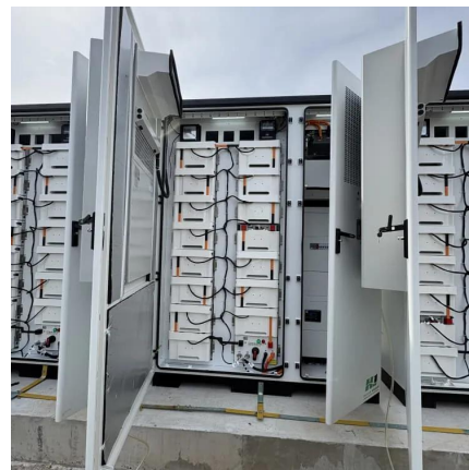
Battery Energy Storage System Container , BESS
